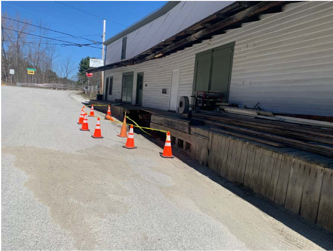
4/24/2026: West River Street drainage issue
